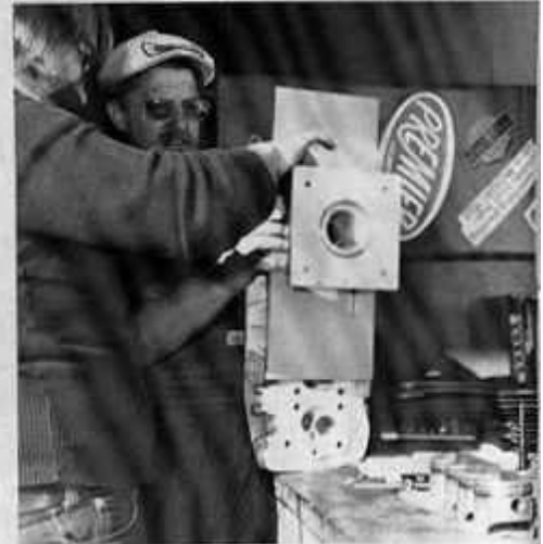
ABOVE—The base part of the flow bench is fabricated to duplicate the flow of air into the cylinder through the port. The most important part of installation is alignment.
